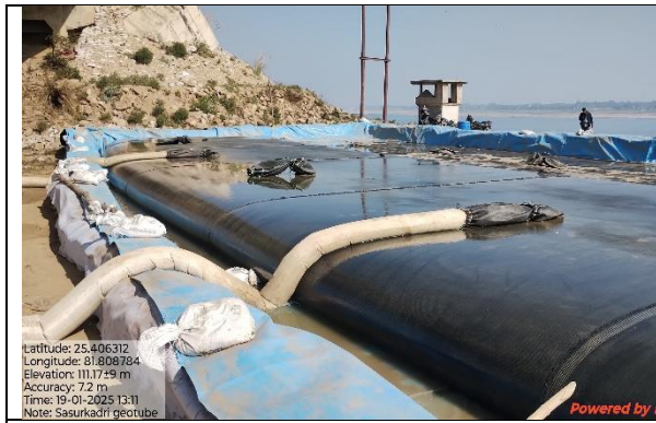
Geosynthetic Dewatering Tubes
