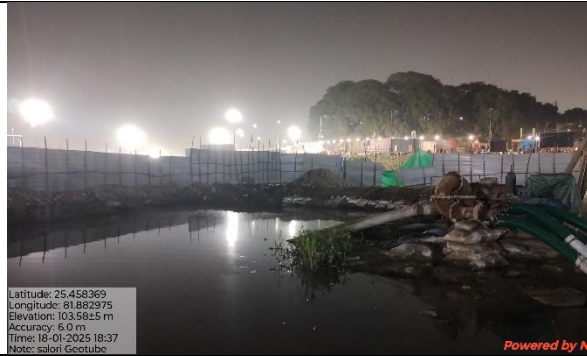
Tapping of Drain for Treatment Through Geo-Tube
